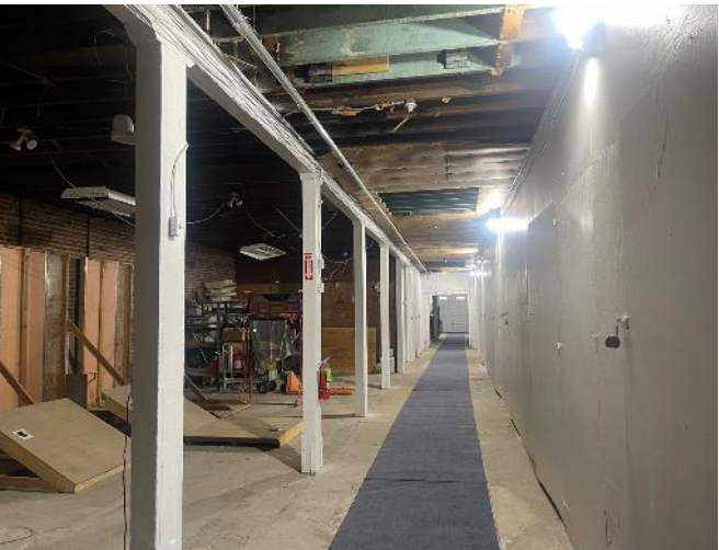
Interior view of the ground floor
